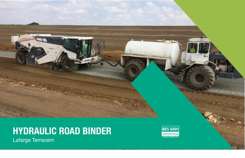
Lafarge Terracem Hydraulic Road Binder is a blend specially formulated for the use in soil stabilisation. Due to this level of blend Lafarge Terracem has lower embodied CO2 than CEM I 52.5N.
